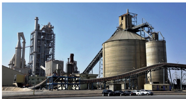
Recycling of drill cuttings at JEL
