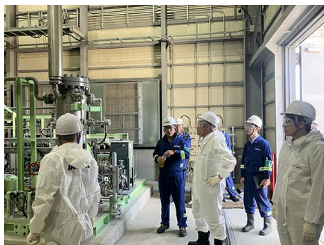
Plant visit at Kashiwazaki Hydrogen Park
