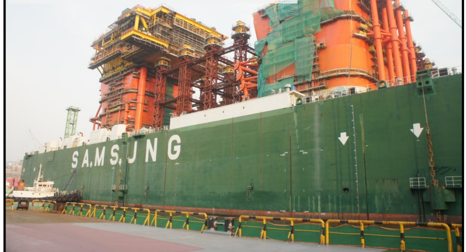
Installation of CPF topside module (April/2015, Korea)
