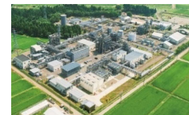
Koshijihara Gas Plant (Niigata, Japan)
