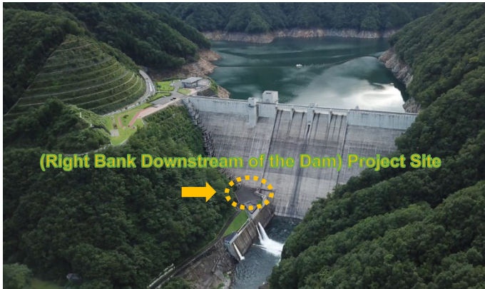
View from Downstream of Yunishigawa Dam
